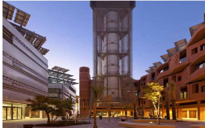
Fig. 15 Roof top PV panels on Masdar institute buildings Reference: http://www.fosterandpartners.com/ , accessed 17 April 2017
