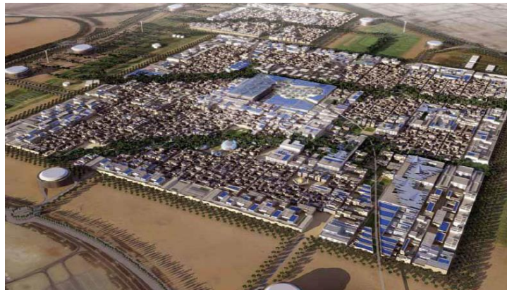
Fig.2 Aerial view of Masdar City, United Arab of Emirates Reference: Stilwel and Lindabury, 2008
